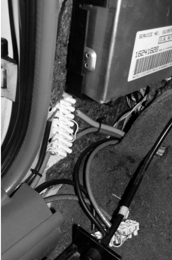
Figure 5.8: Inside cab, passenger's side. View laser cables, which are run beneath plastic liner below door, laser cable junction boxes, throttle actuator, ...?
