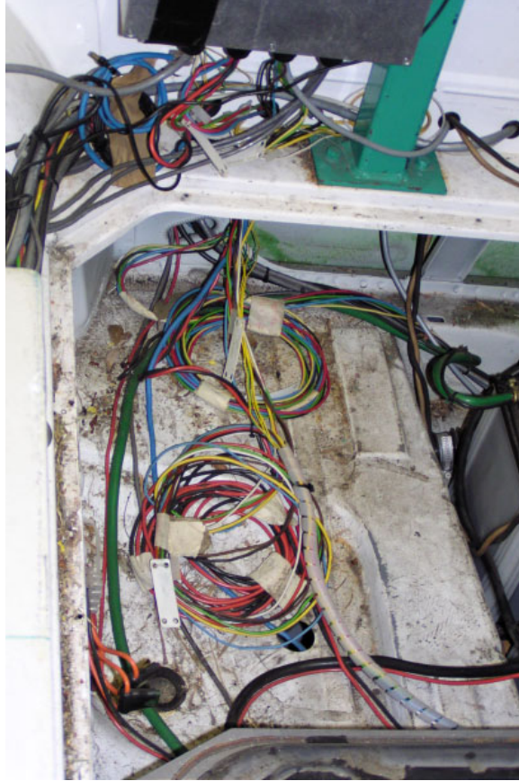
Figure 5.2: Cables run beneath the tray (accessible via cover) to the cab.
